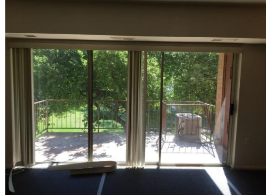
Figure 35: Typical Balcony Door
