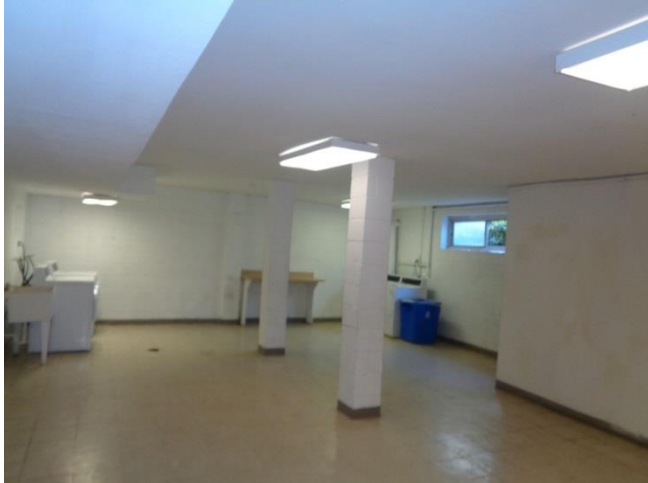
Figure 16: Typical Laundry Fixtures
