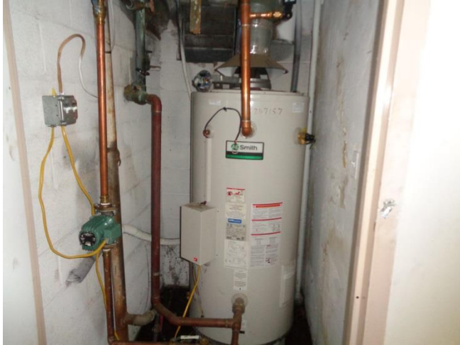
Figure 14: Typical Domestic Hot Water Heater
