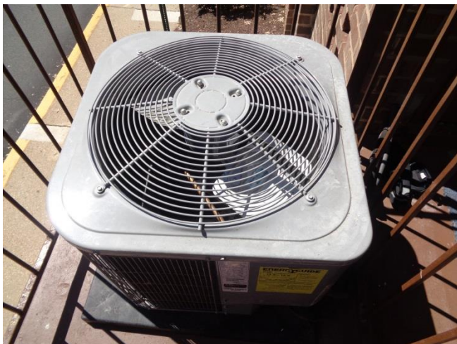
Figure 8: Typical Condensing Unit for Apartments
