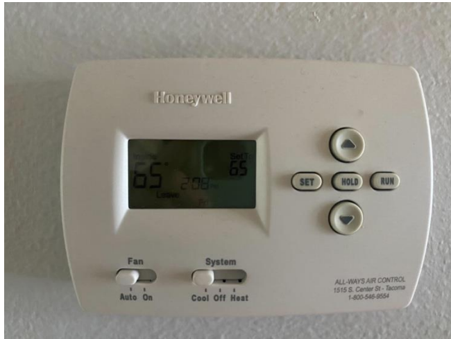
Figure 12: Typical Furnace Thermostat
