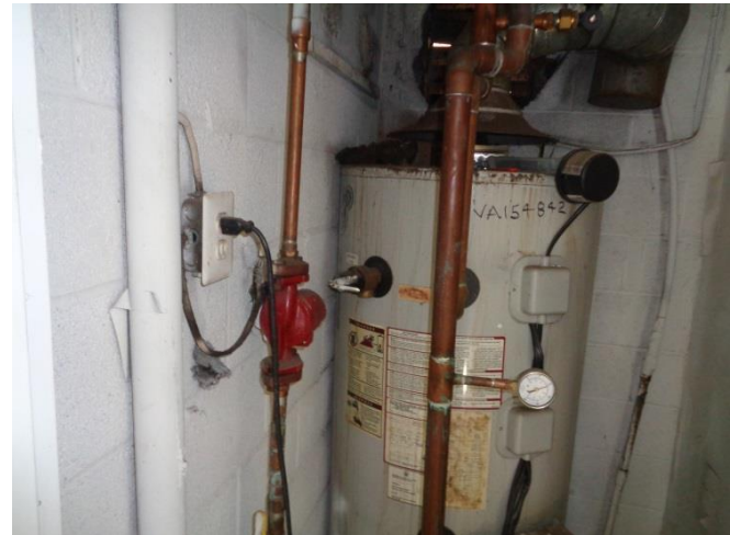
Figure 42: Typical DHW Piping
