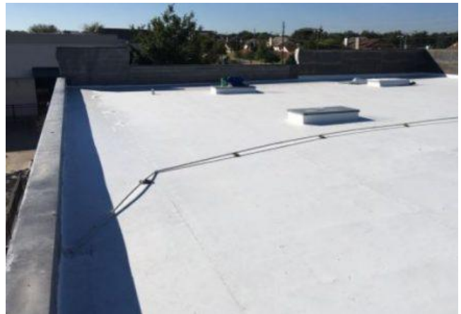
Figure 33: Typical Rooftop View
