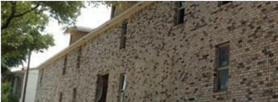
Heroes House in Dallas, part of the HOME Investment Partnership Program. Source: heroeshousetx.com
